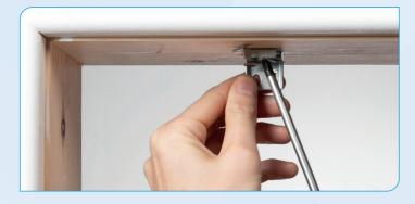
B. Carefully screw each bracket into place, ensuring they are aligned with one another in a straight row.
