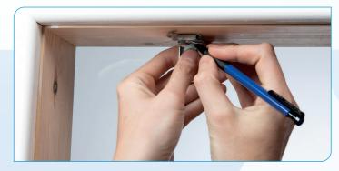
A. Using one of the brackets as a template mark up the first hole with a pencil. Repeat this, taking into consideration that the brackets should be spaced out at equal intervals. Once all positions have been marked, drill holes in each position. If required, fit wall plugs.
